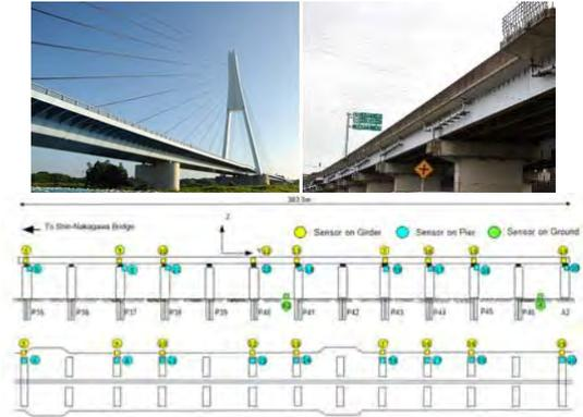
Fig. 4. Shin-Nakagawa (top left) & Katsuta Bridge (top right), Wireless monitoring system of Shin-Nakagawa and Katsuta Viaduct (bottom).
