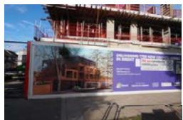
写真1:Preston Community Library (改築中)
